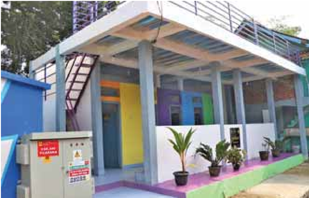
Newly-constructed sanitation facilities in a pesantren 5
